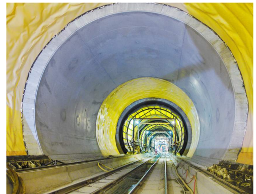
Cast-in-Place Lining
